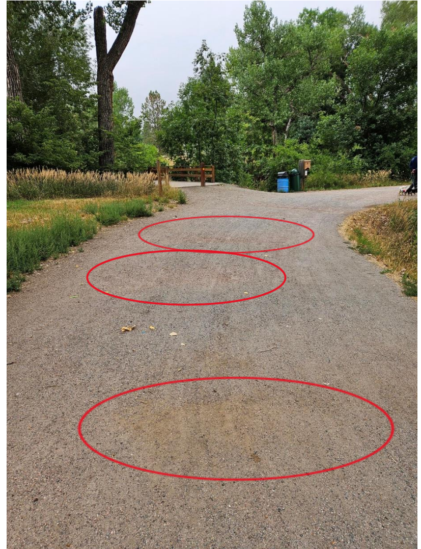
Dirt showing through the trail surface where the crusher fines have worn away
