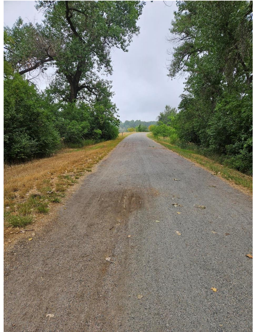
Ruts and dirt showing through where the trail surface is worn out
