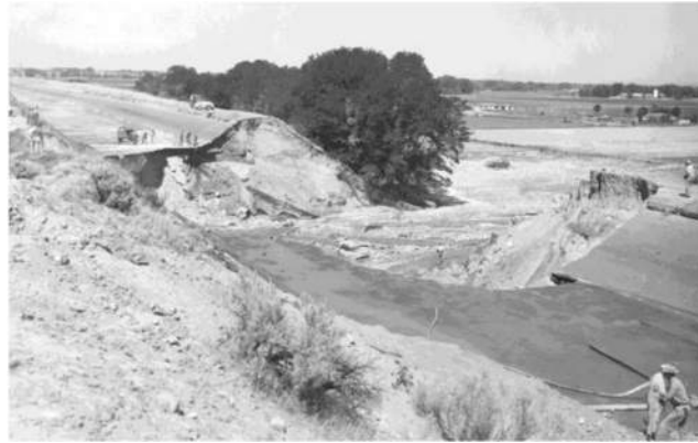
Figure 2 - USBR, example ditch embankment failure
